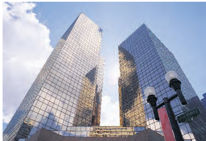
The Scotia Place twin office towers, 28 and 21 stories respectively, stand prominently in the center of Edmonton's downtown commercial and retail properties.
